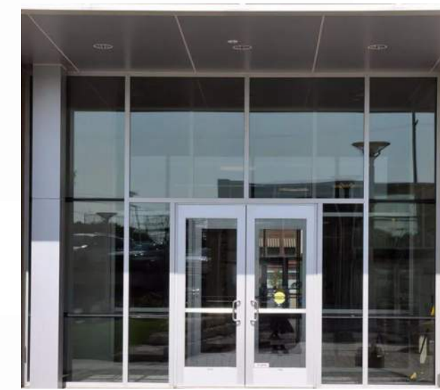
STF-01 Storefront System (with Doors in Entry)
