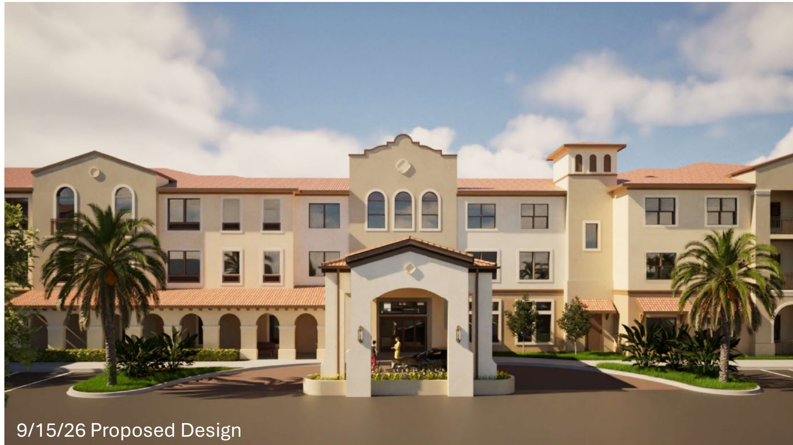
Front (South) Elevation Close-up
