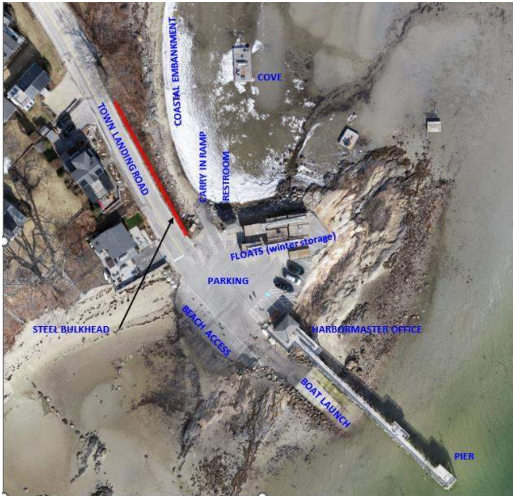
Fig. 2. Falmouth Town Landing Facilities- GEI Drone Photo Composite (2022)
