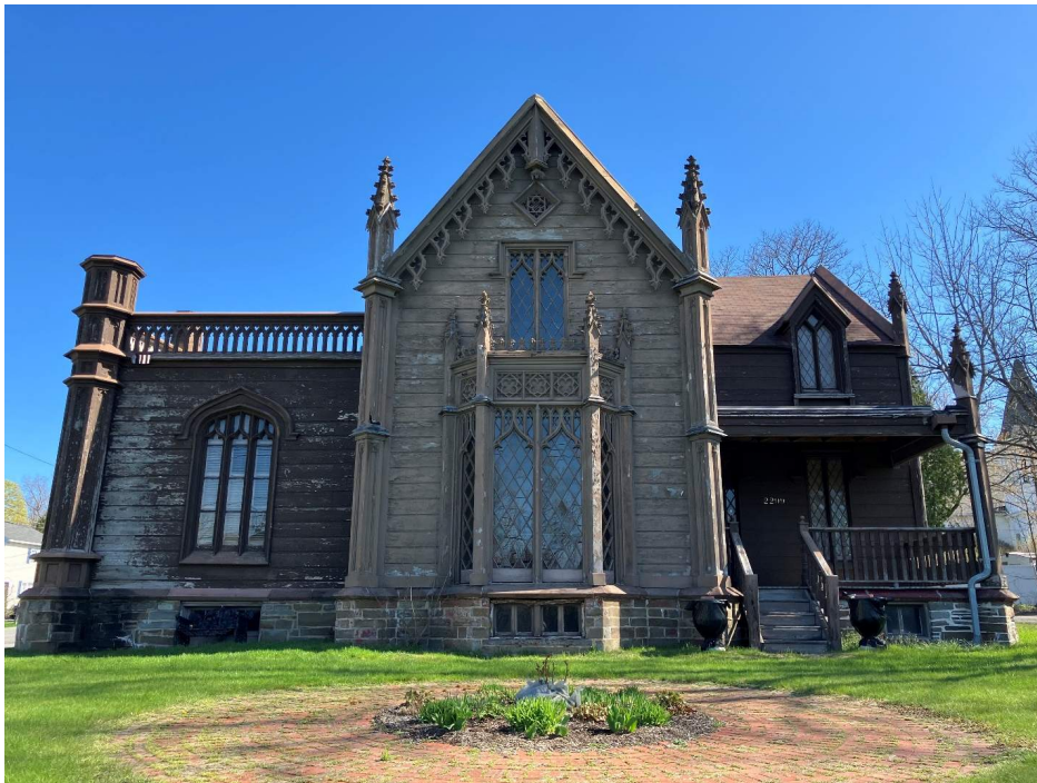
The Schoolcraft House (circa 1840), located on Western Avenue near the Guilderland Fire Department Station, is slated for renovations to improve its appearance and accessibility.
