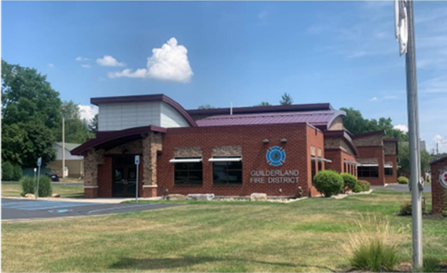
Guilderland Fire District building at 2303 Western Avenue
