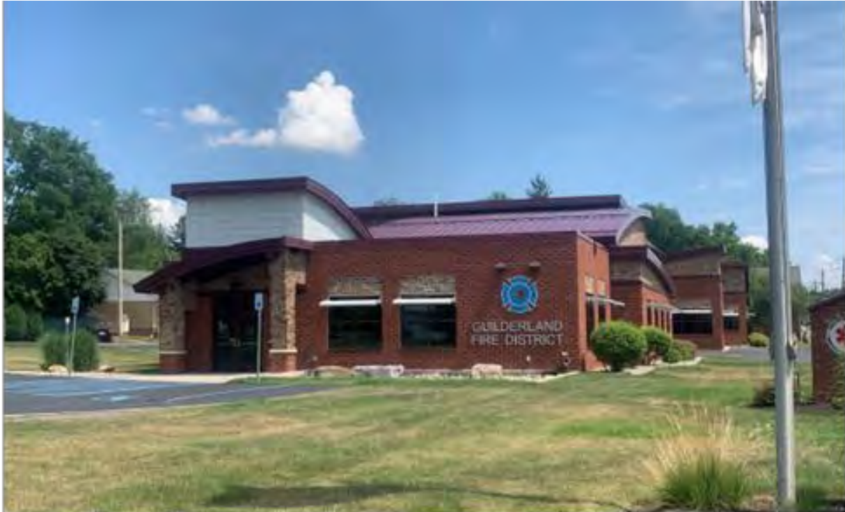
Guilderland Fire District building at 2303 Western Avenue
