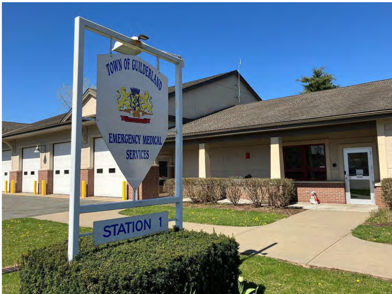
Town of Guilderland Emergency Services Station 1 building in Westmere
