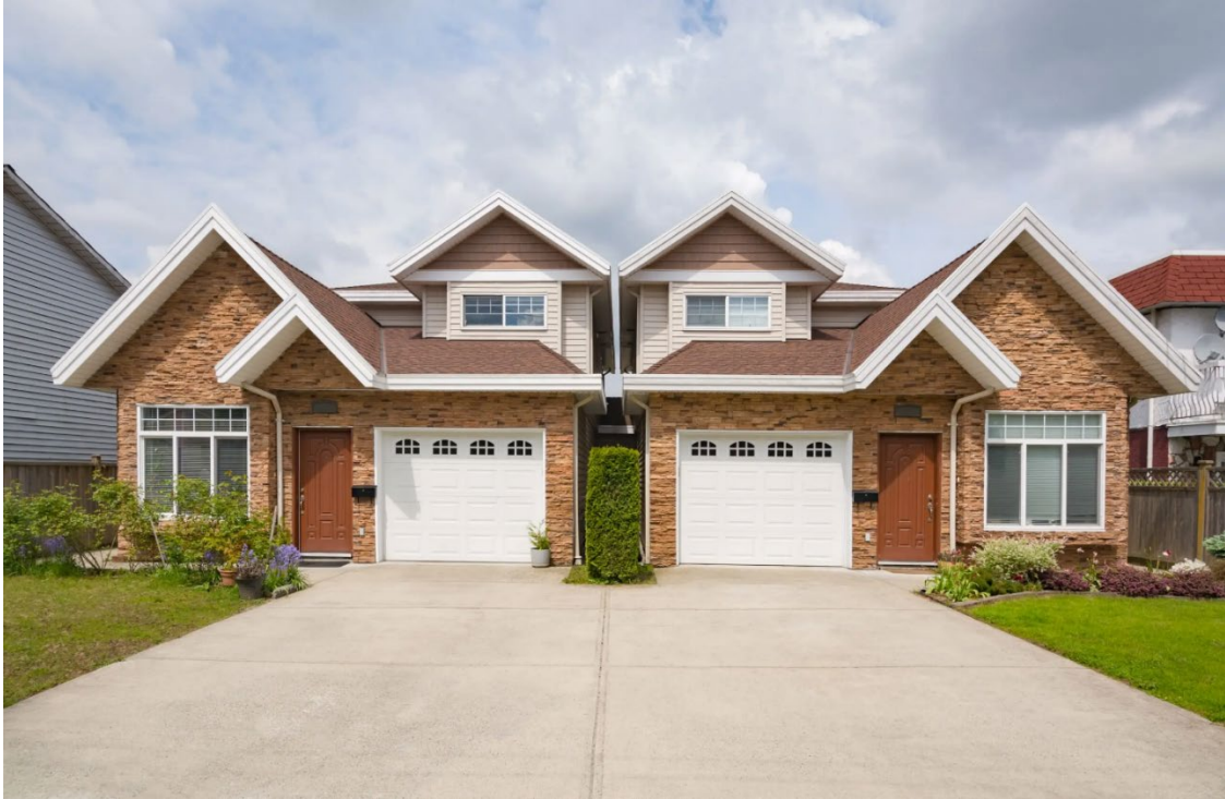
An example of a side-by-side 2-family dwelling with dimensional standards comparable to a single-family dwelling. Photo courtesy of: www.newwestern.com/blog/cost-to-build-a-duplex/
