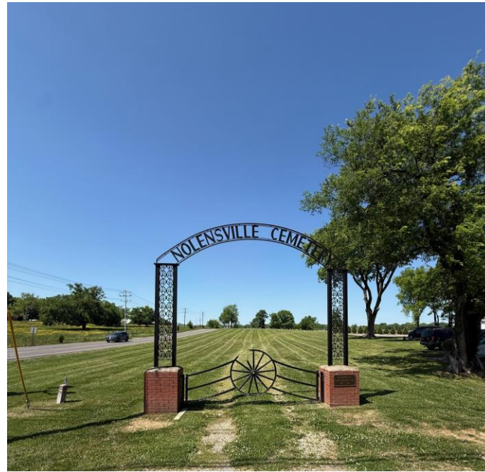
Existing Archway Facing Nolensville Road
