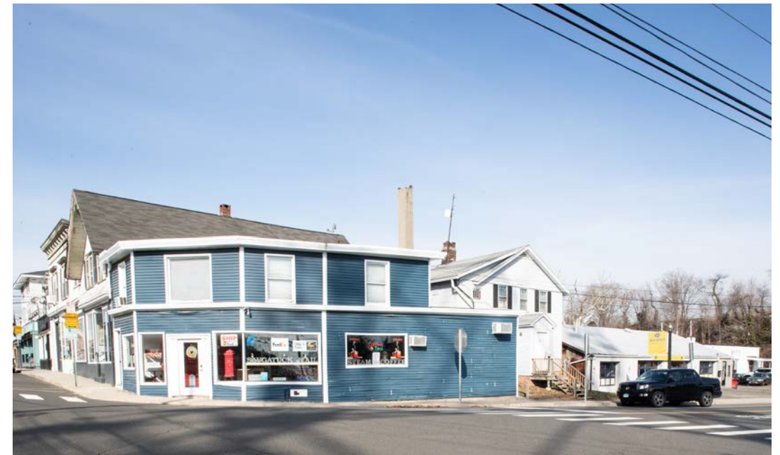
Corner of Riverside and Railroad Place
