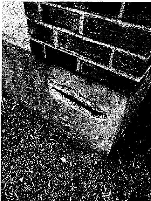
Spalled section at the southeast corner:
