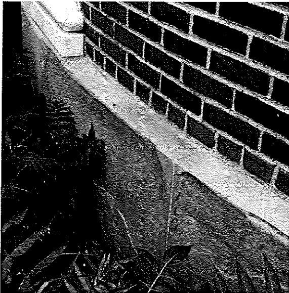
Spalled section at the southeast corner:
