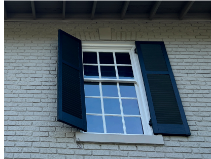
Existing Operable Shutters
