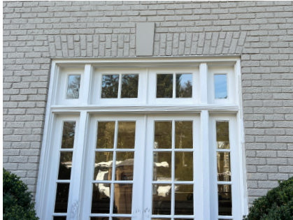
Existing Window/Door Header
