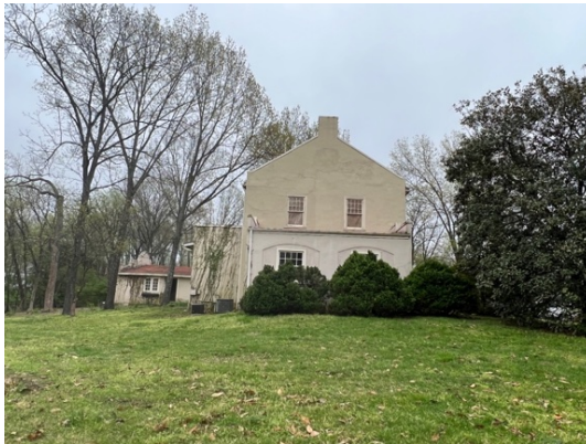
Side (Facing Jackson Blvd.)- 4424 Shepard Place
