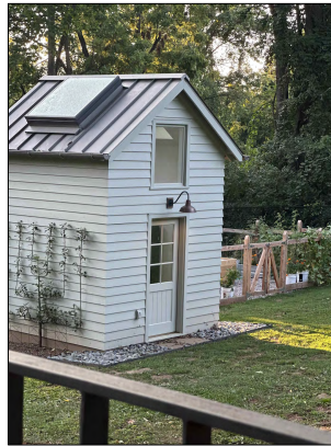
11-2 PAINTED CEDAR SIDING, BONDERIZED STEEL ROOF & GUTTERS
