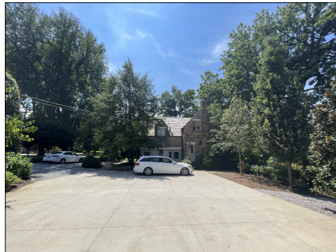
3 REAR OF RESIDENCE DUKE HZC 08-16-2024
