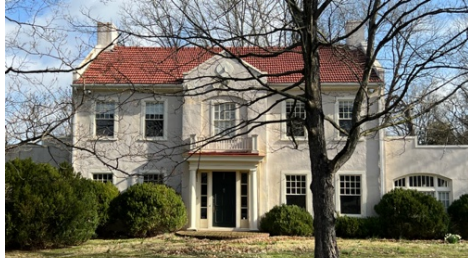
Exhibit A: Red clay roof tiles to remain
