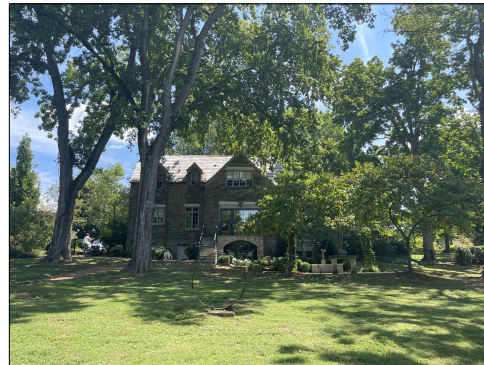
4 NORTH SIDE OF RESIDENCE DUKE HZC 08-16-2024
