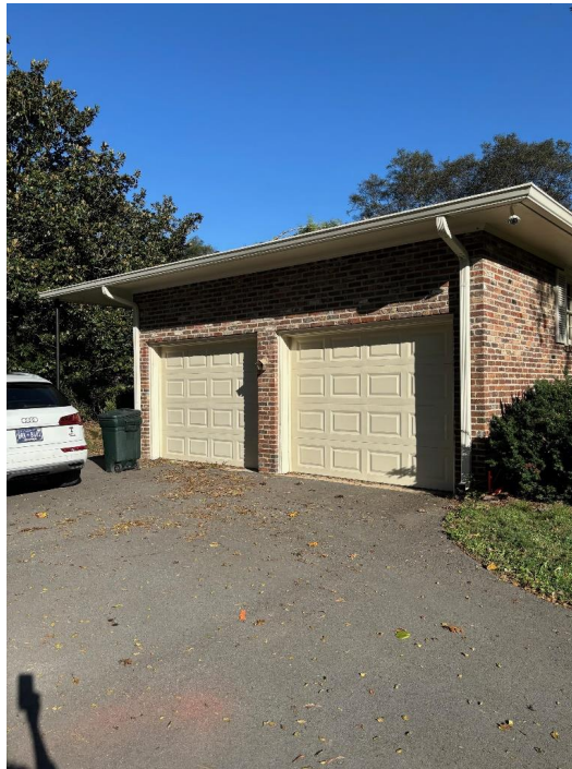
LOCATION OF REAR LEFT CORNER OF NEW GARAGE (ORANGE TAG ON DRIVE)
