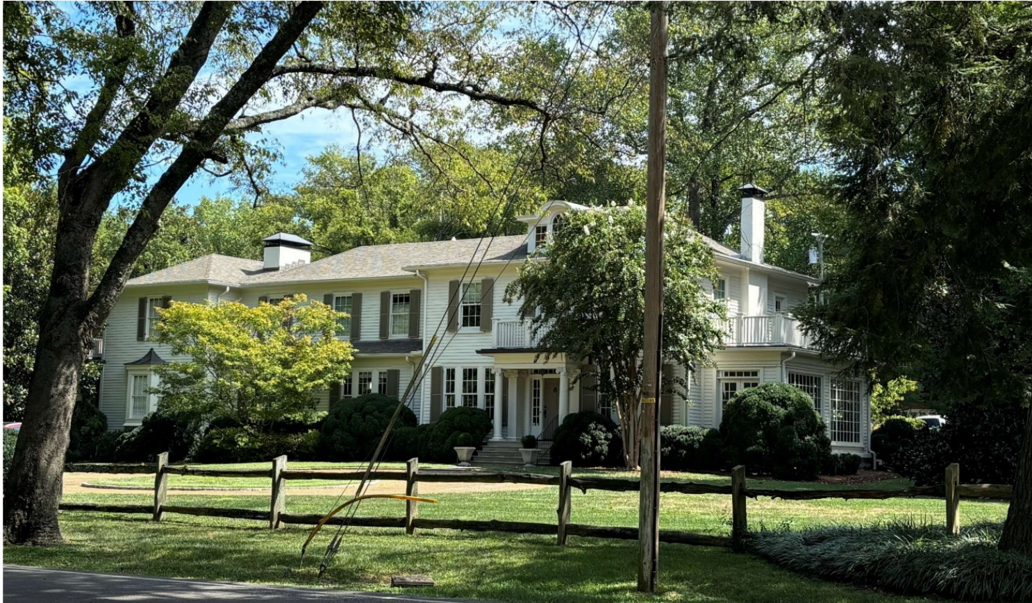
Nesbitt Residence 224 Lynnwood Boulevard Nashville, TN (Belle Meade)
