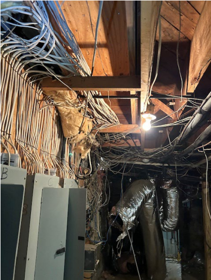
Crawlspace of Original (Amount of Renovation Evidence)
