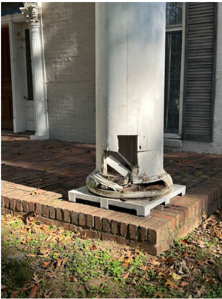
Original Porch Support Column
