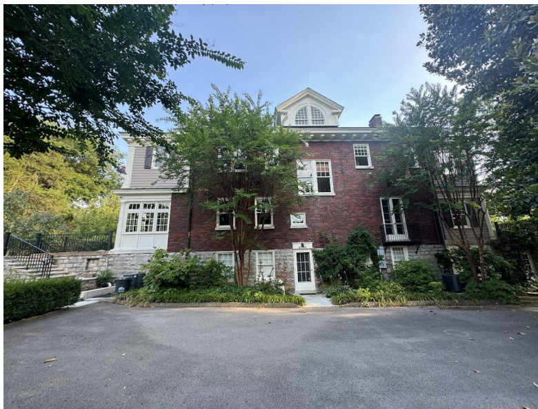
EXISTING REAR OF HOUSE
