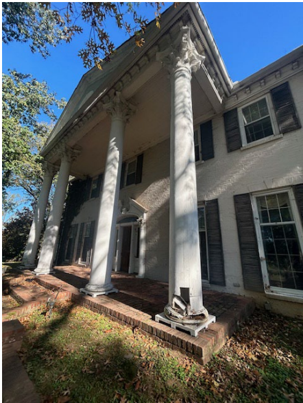
Original Porch Support Column
