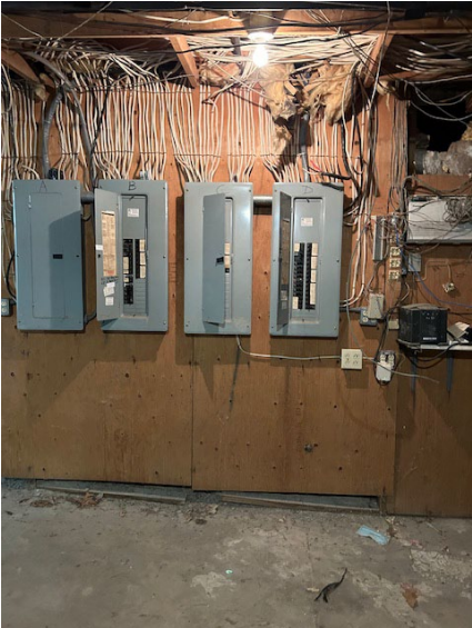
Crawlspace of Original (Amount of Renovation Evidence)
