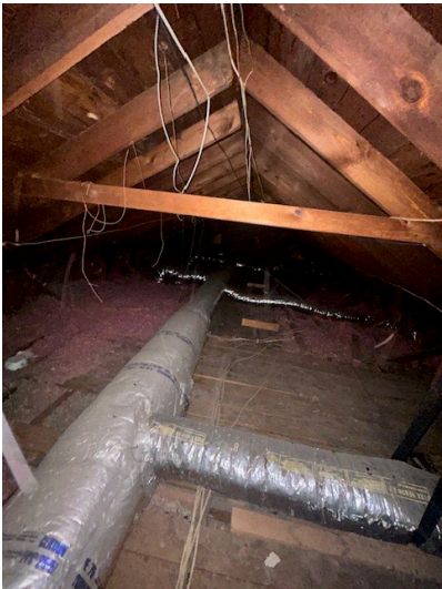
Original Attic Framing
