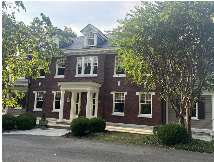
EXISTING FRONT OF HOUSE
