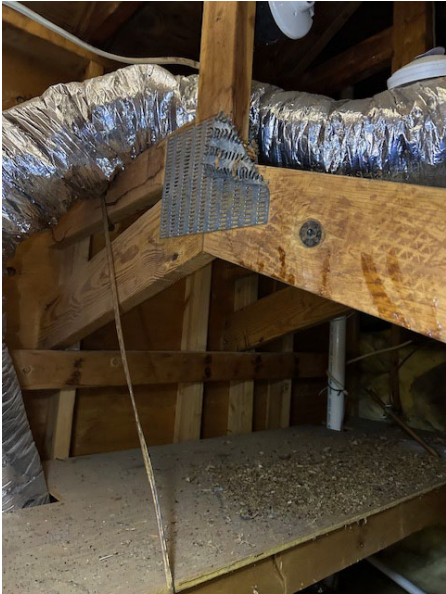
Addition Attic Framing
