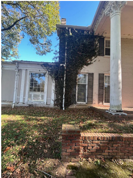
Original Porch Support Column
