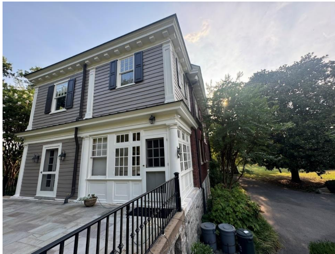
EXISTING RIGHT SIDE OF HOUSE
