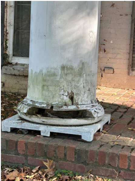
Original Porch Support Column
