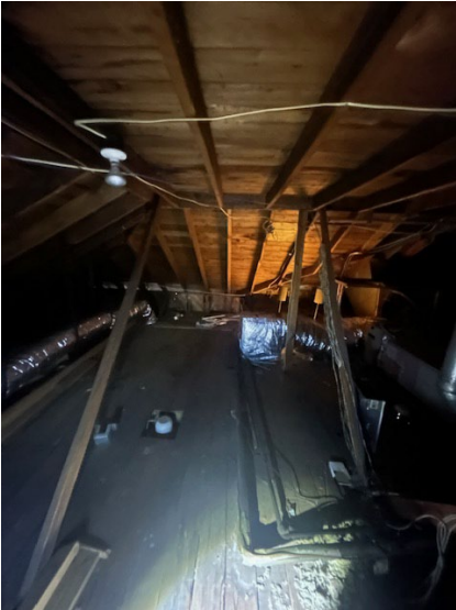
Original Attic Framing
