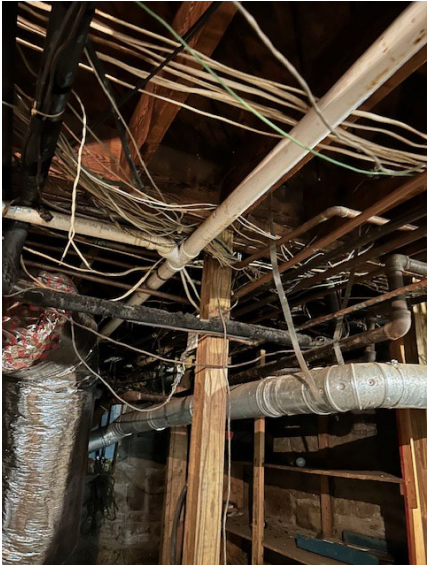
Crawlspace of Original (Amount of Renovation Evidence)
