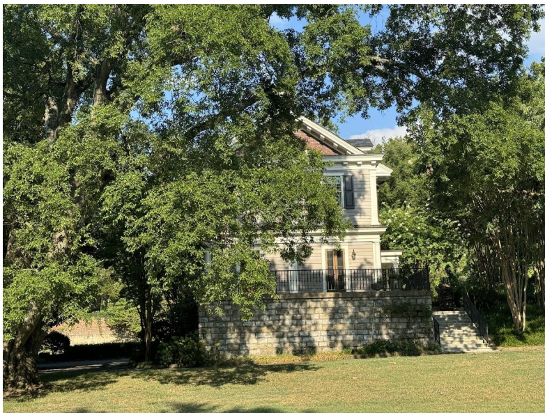
EXISTING LEFT SIDE OF HOUSE
