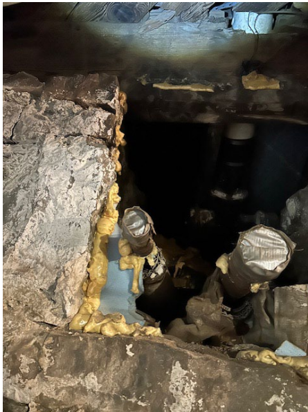
Crawlspace of Original
