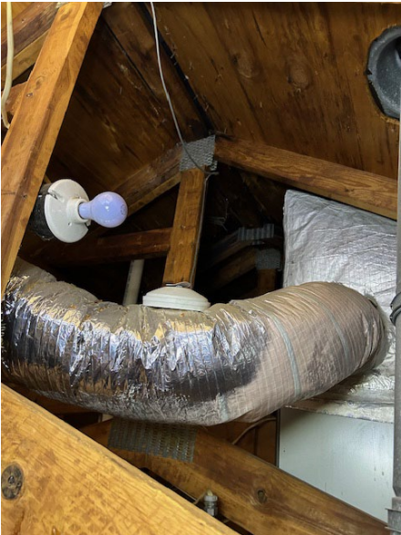
Addition Attic Framing
