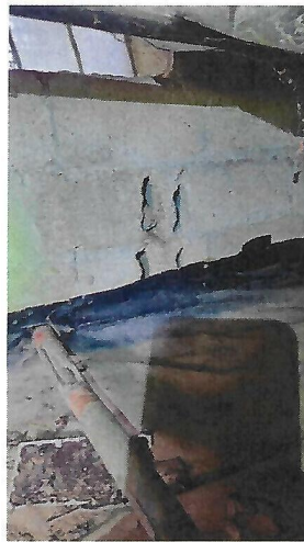
Crawlspace - Significant Water Intrusion, Structural Cracking - At Addition Crawl Space, Very Short Access and Filled with Water.
