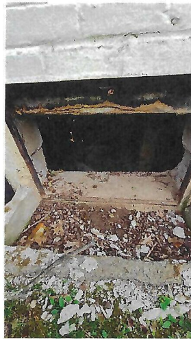
Crawlspace - Significant Water Intrusion, Structural Cracking - At Addition Crawl Space, Very Short Access and Filled with Water.
