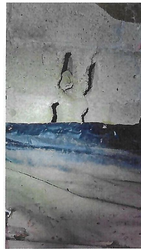
Crawlspace - Significant Water Intrusion, Structural Cracking - At Addition Crawl Space, Very Short Access and Filled with Water.
