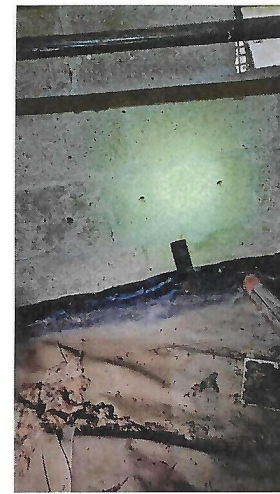
Crawlspace - Significant Water Intrusion, Structural Cracking - At Addition Crawl Space, Very Short Access and Filled with Water.
