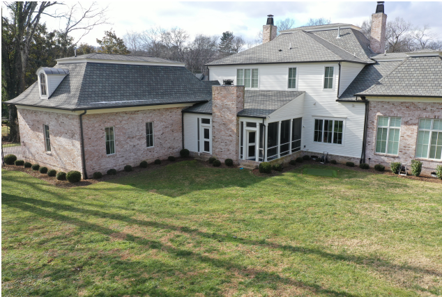
Existing Rear of House
