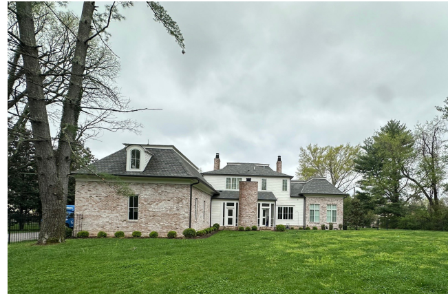
Existing Rear of House
