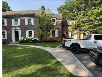
2 site photo not for scale
