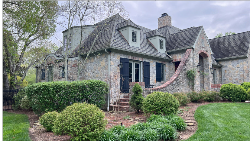
4430 E BROOKFIELD | EXISTING | PRIMARY SUITE
