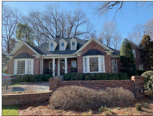
VIEW OF THE STREET FACADE FROM THE EAST
