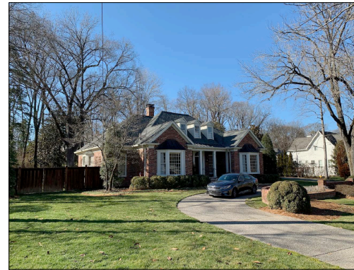
VIEW OF THE STREET FACADE FROM THE EAST
