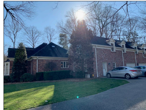
VIEW OF THE NORTH ELEVATION
