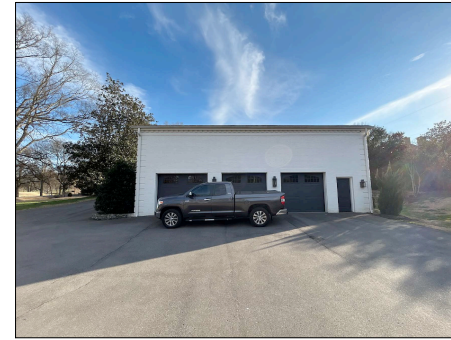
VIEW OF THE NORTH ELEVATION
