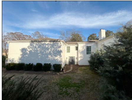
VIEW OF THE PARTIAL WEST ELEVATION
