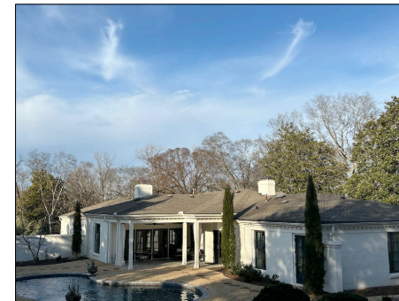
VIEW OF THE SOUTH ELEVATION FROM THE SOUTHWEST
