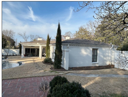
VIEW OF THE SOUTH ELEVATION
