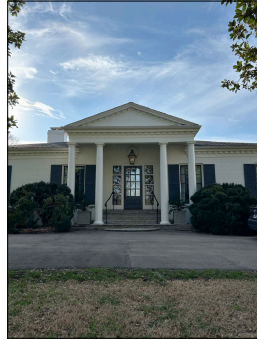
VIEW OF THE FRONT FACADE FROM THE STREET
