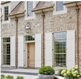
GUTTERS COPPER GUTTERS & DOWNSPOUTS
