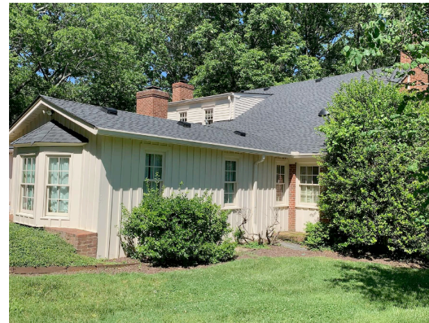
VIEW OF THE SIDE FACADE FROM THE SOUTH-WEST
