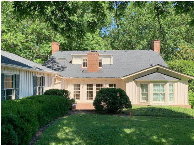
VIEW OF THE REAR FACADE FROM THE WEST
