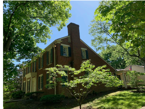
VIEW OF THE SIDE FACADE FROM THE NORTH
