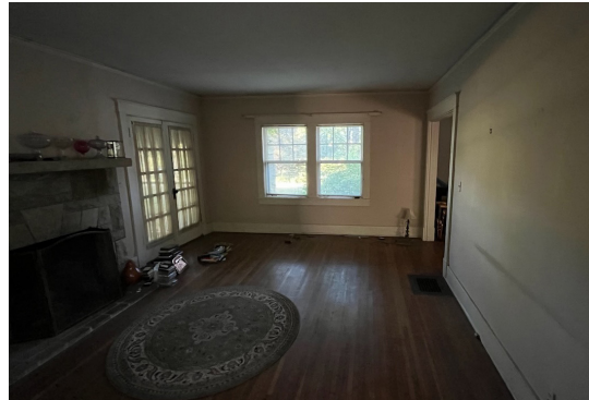
Typical Interior Condition - Main Floor
