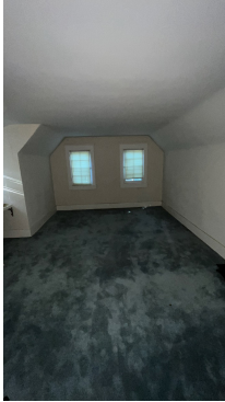
Typical Upper Floor Room - Low Ceiling.
