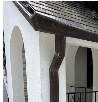
Gutters: Gutters to match existing
