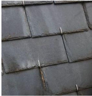
Slate Roofing: Slate to match existing
