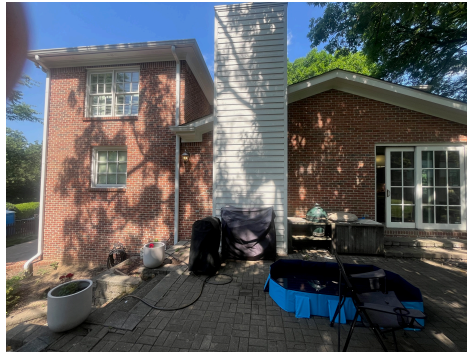
rear of house
