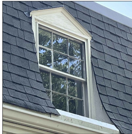
existing asphalt shingle roof
