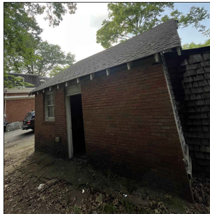
shed/storage side entry - proposed to be demolished
