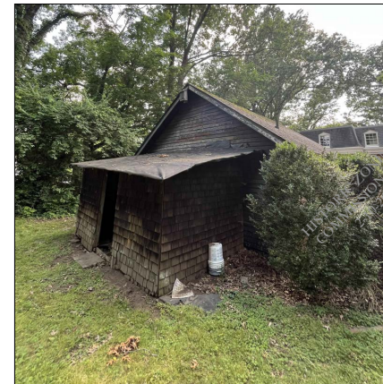
storage/shed rear - proposed to be demolished
