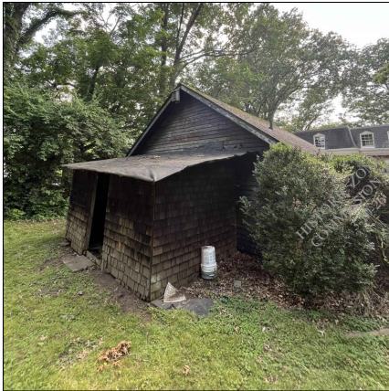
storage/shed rear - proposed to be demolished
