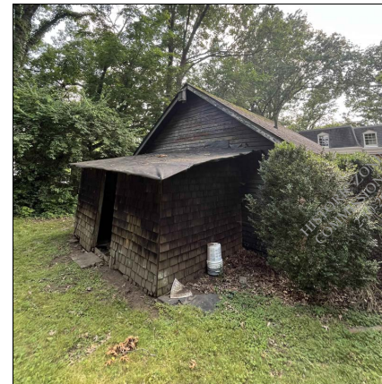
storage/shed rear - proposed to be demolished
