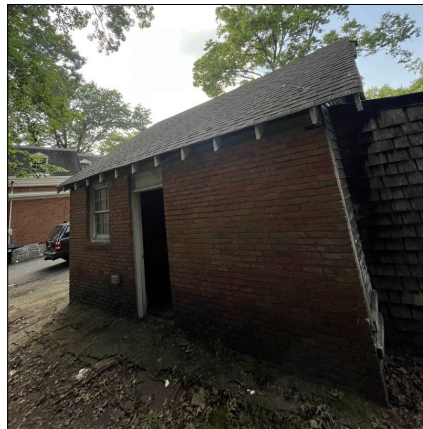
shed/storage side entry - proposed to be demolished
