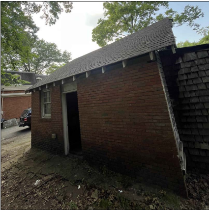
shed/storage side entry - proposed to be demolished
