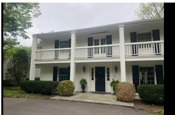
FRONT OF EXISTING HOUSE
