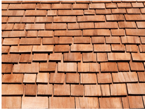
cedar shake roof
