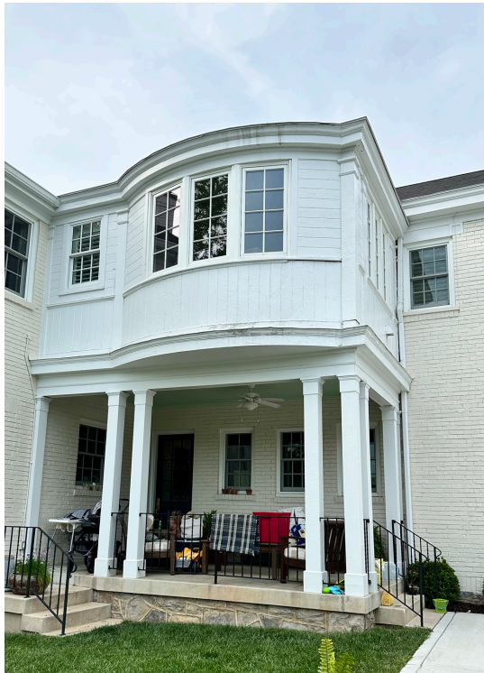
Wood Porch to be Demolished - Rear View
