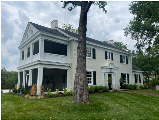
Current Front Facade
