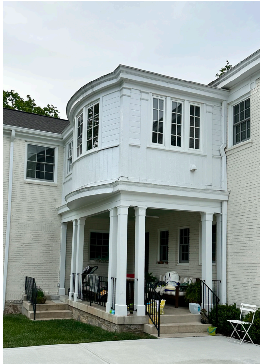
Wood Porch to be Demolished - Side View
