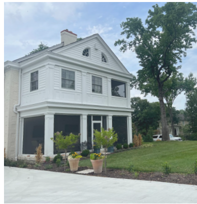
Current Side Facade
