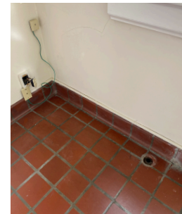
Interior Floor Condition of Porch
