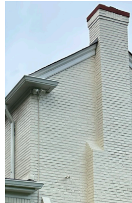
Painted Brick Chimney
