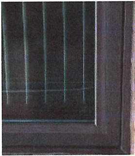
dark bronze windows and gutters
