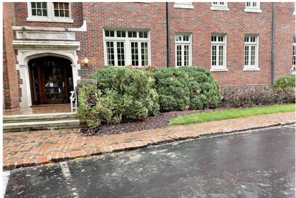
1 Z5.1 brick walk at left front entrance
