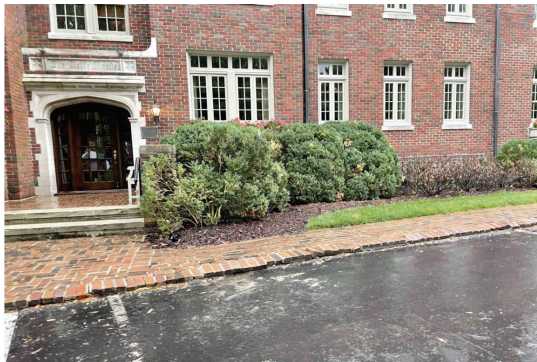
1 Z5.1 brick walk at left front entrance
