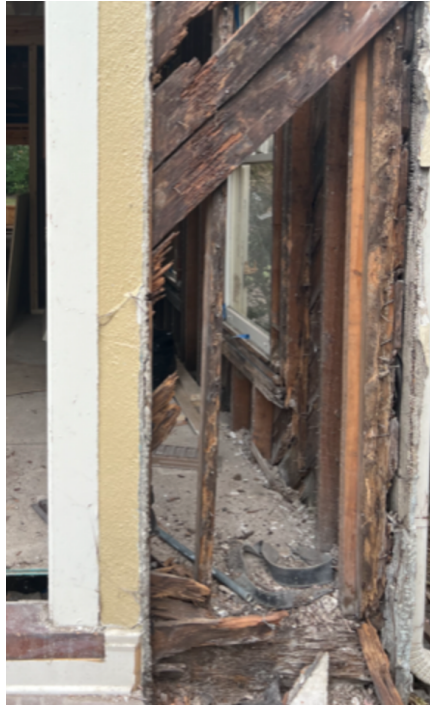
E. Side Façade (Jackson Blvd.)
