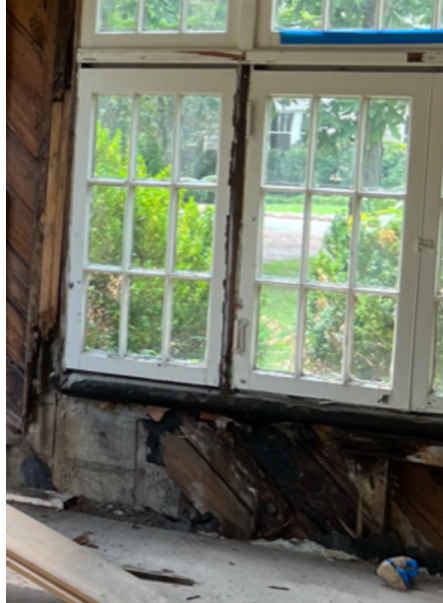
B. Rear and Side Façade (Jackson Blvd.)-Exposed gap lacking any material coverage between interior and exterior. Exposed "patch" from previous home owner during window retrofit. Patched gaps (roughly 18" x 60" in 12 separate locations on all exterior walls).
