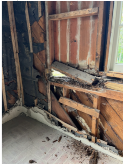
B. Rear and Side Façade (Jackson Blvd.)-Exposed gap lacking any material coverage between interior and exterior. Exposed "patch" from previous home owner during window retrofit. Patched gaps (roughly 18" x 60" in 12 separate locations on all exterior walls).
