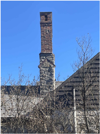
Ⓒ Existing Brick Chimney
