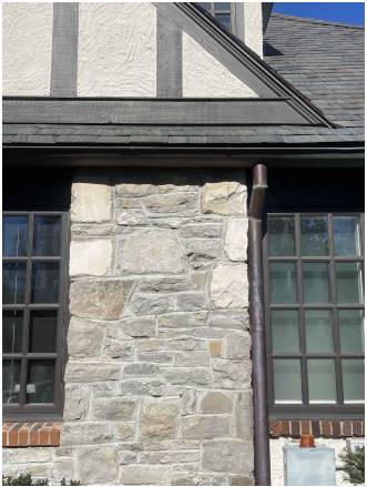
Ⓑ Existing Stone Facade & Wood Trim
