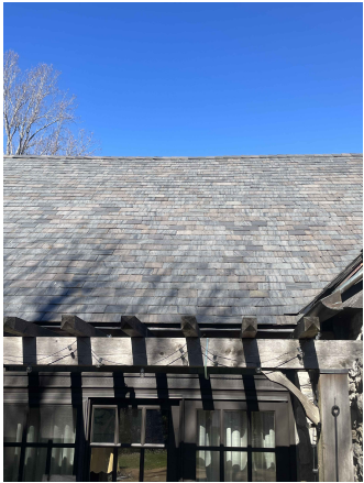
Ⓐ Existing Slate Roof
