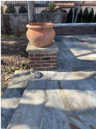
Ⓔ Existing Terrace Pavers & Brick Landscape Wall
