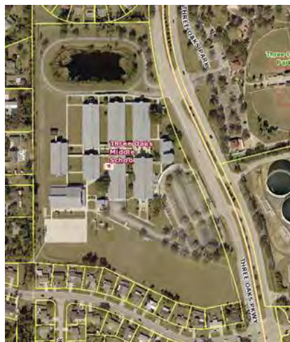
Figure 3: Aerial of Three Oaks Middle School
