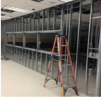
Collier County Schools Continuing Contract Renovation project for Collier Schools
