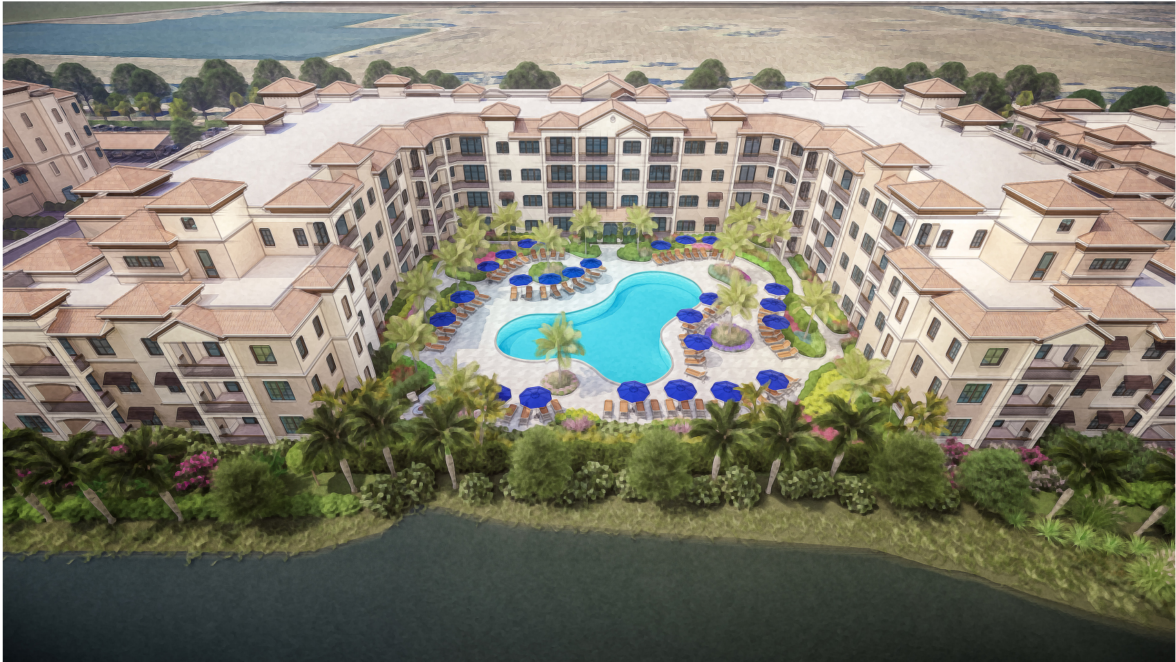
BUILDING B AMENITY DECK
