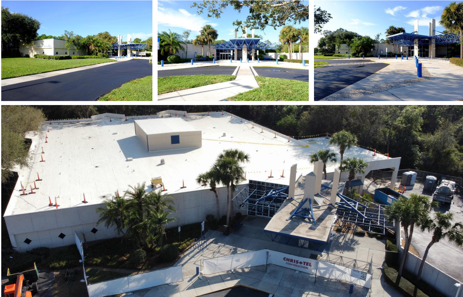
GRACE HEBERT CURTIS ARCHITECTS SOUTH COUNTY REGIONAL LIBRARY | 02.28.2025 CURRENT EXISTING CONDITIONS
