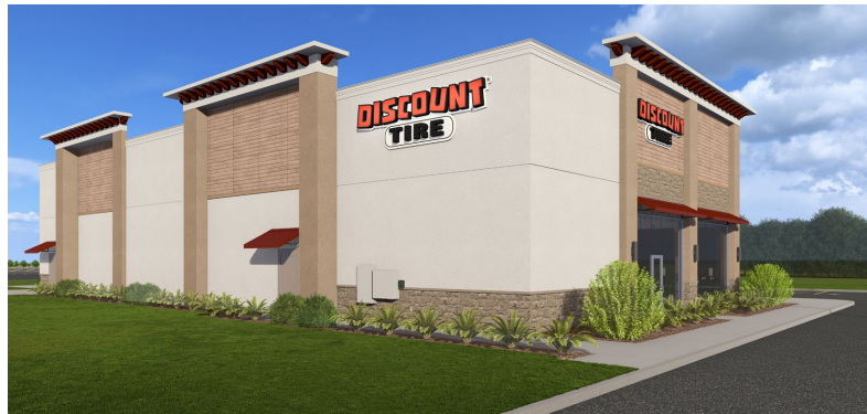
SIDE ENTRANCE VIEW
