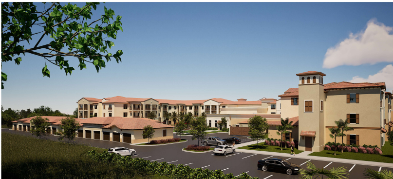
View 1 - Northwest (Rear) Corner Elevation
