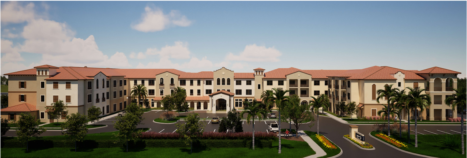
View 1 - South (Front) Elevation
