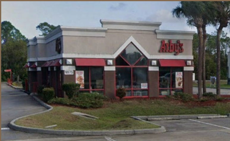
Existing Front Façade
