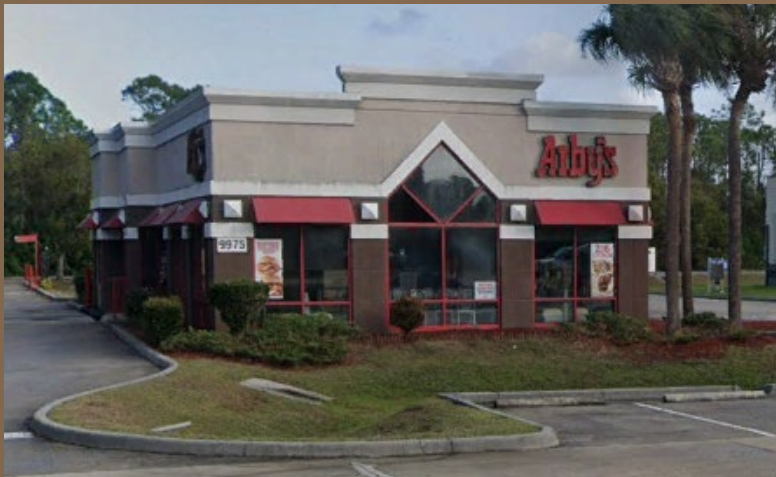
Existing Front Façade
