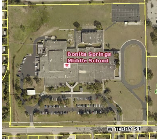
Figure 4: Aerial of Bonita Springs Middle School
