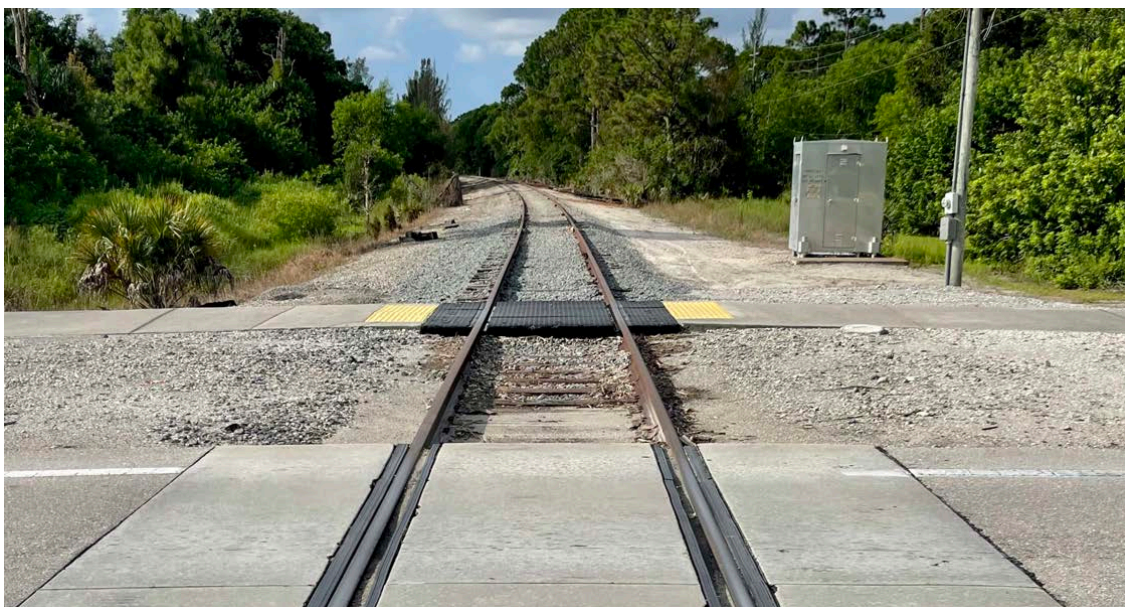
Rail crossing at Corkscrew Road looking north
