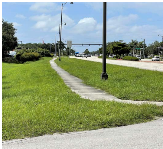
US Highway 41 looking south at Old 41 Road
