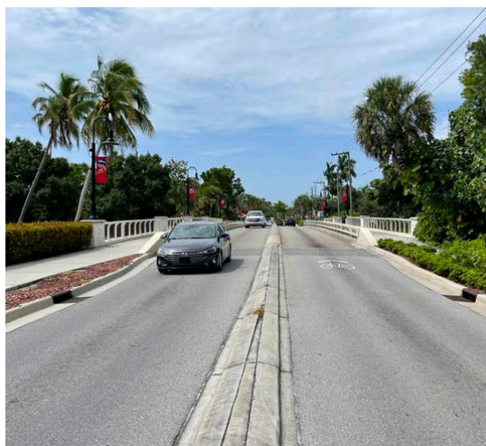
Old 41 Road crossing Imperial River
