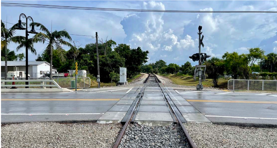
Rail crossing East Terry Street
