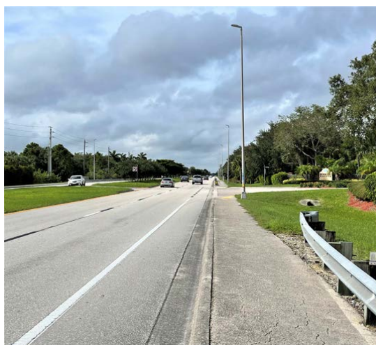
South of Estero Road on Three Oaks Parkway looking South
