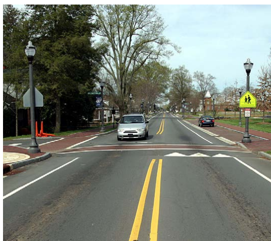
Marked and signed crossing in Cornelius, North Carolina
