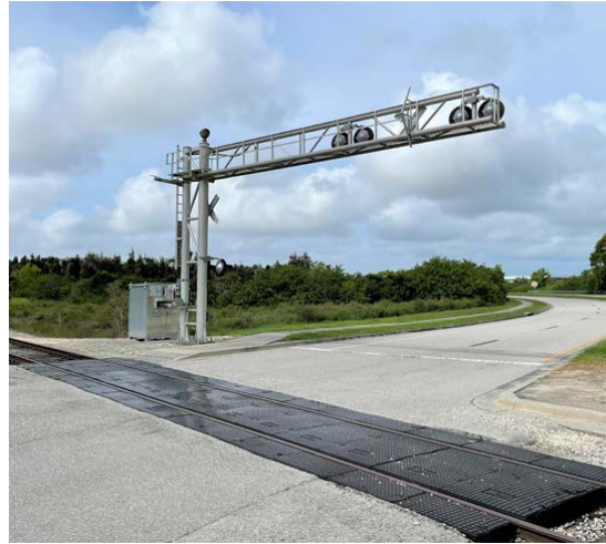
Rail crossing at Coconut Road looking southwest
