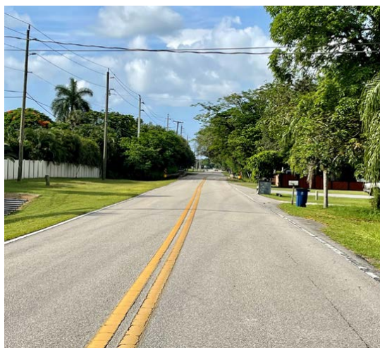
Sandy Lane looking South
