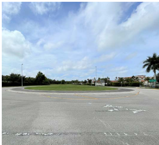
Via Coconut Road roundabout looking south toward Production Boulevard
