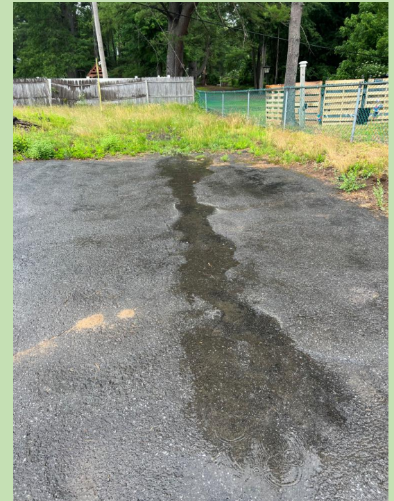
Drainage during rain event, flowing towards proposed retention basin
