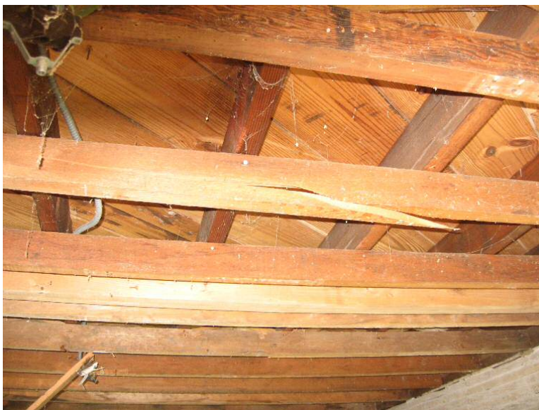
Figure 2. Failure of wood lower 'joist' due to deflection.
