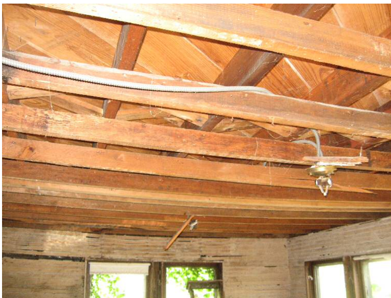
Figure 1. Excessive permanent bowing in floor above.
