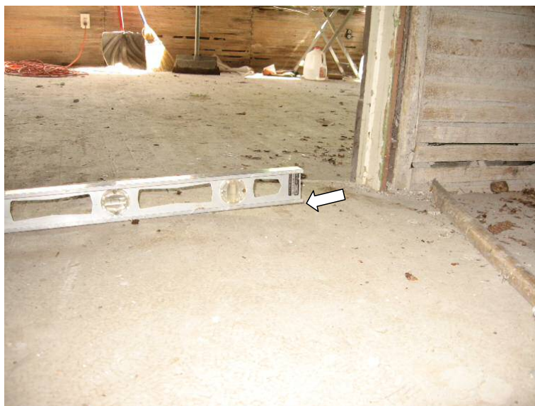
Figure 4. Bowed floor (arrow indicates \frac{1}{2} " gap).
