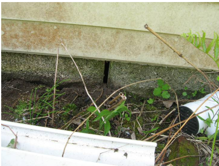
Figure 5. Gap of missing mortar and/or CMU separation.
