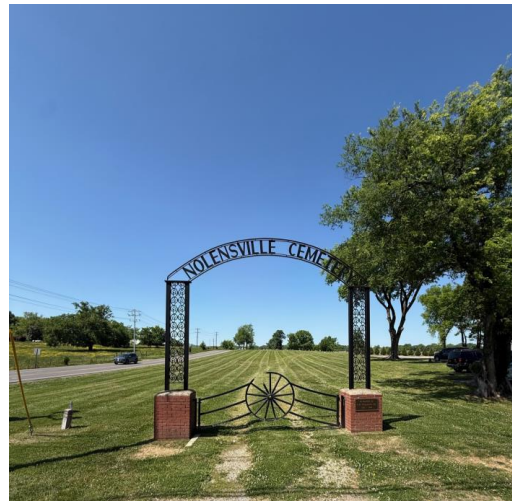
Existing Archway Facing Nolensville Road
