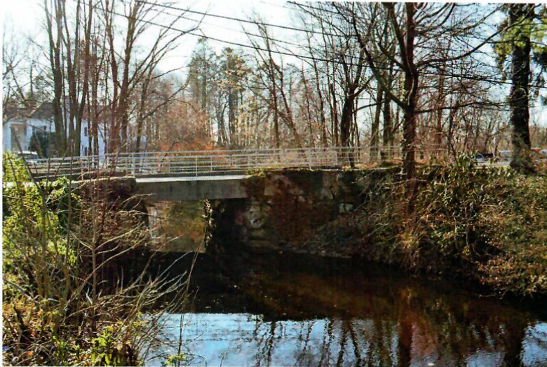
View looking north at south face of bridge.
