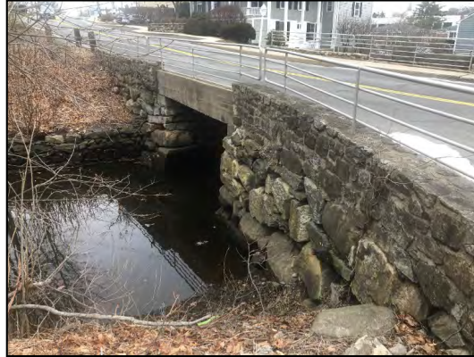
Figure 4: Jesup Road Bridge South Side Looking NW
