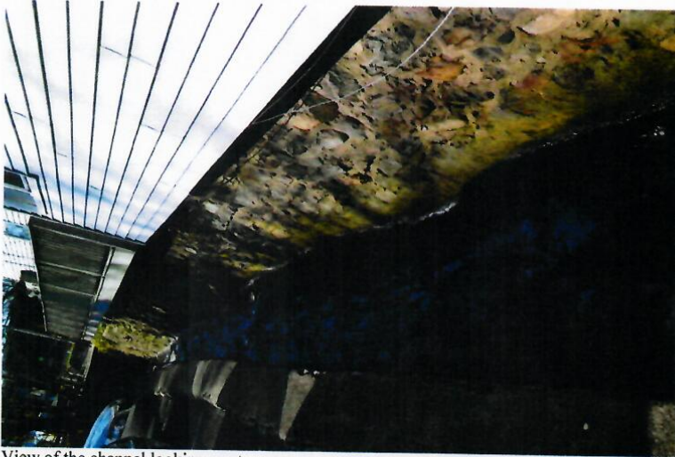
View of the channel looking west.
