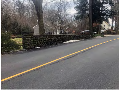
Figure 1: Evergreen Avenue Bridge - South Parapet Wall Looking SW
