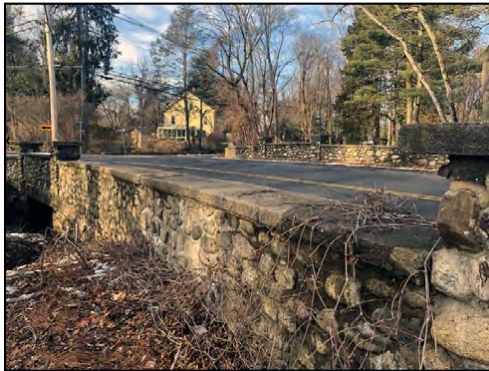
Figure 5: Greens Farms Road Bridge – South Parapet Wall Looking NW
