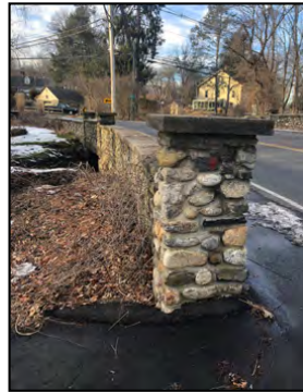
Figure 6: Greens Farms Road Bridge – View of Post at East Side Looking NW
