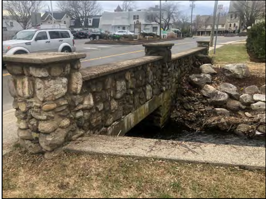
Figure 11 - Myrtle Avenue Bridge North Parapet Wall Looking SW
