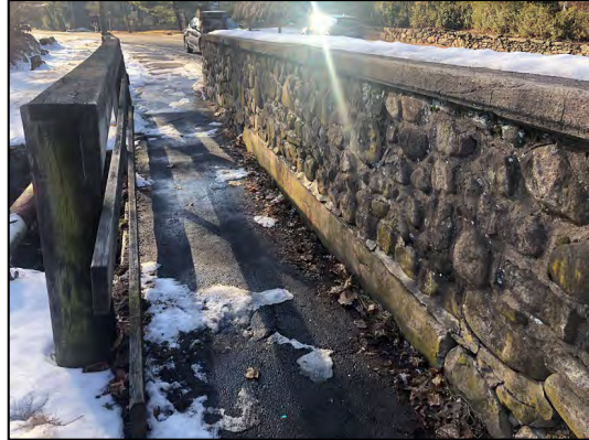
Figure 10 – Long Lots Road - View of South Parapet Wall Looking W
