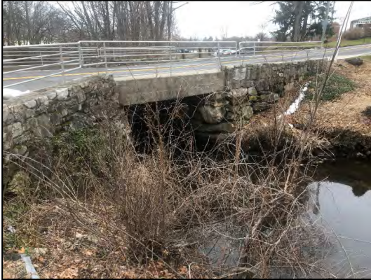
Figure 3: Jesup Road Bridge North Side Looking SW
